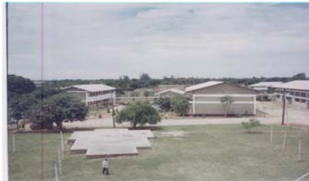
Cross section of Mtwara Regional Vocational Training and Service Centre buildings financed through SDL
