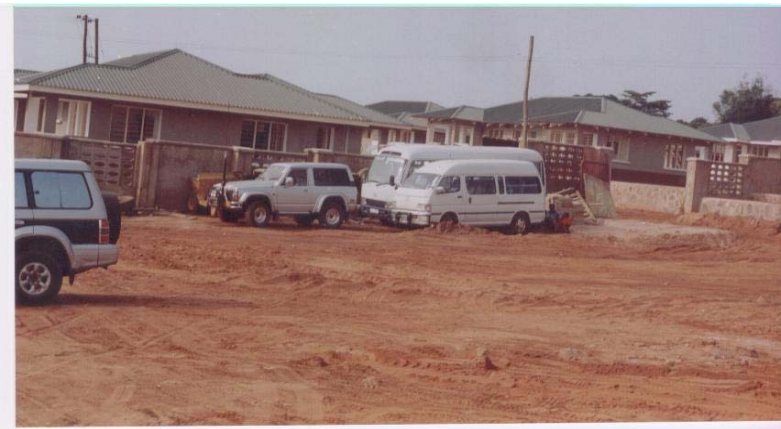
View of Kigoma RVTSC at Mlole area
